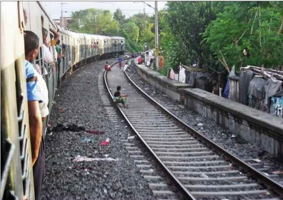
Under construction Tangra station
