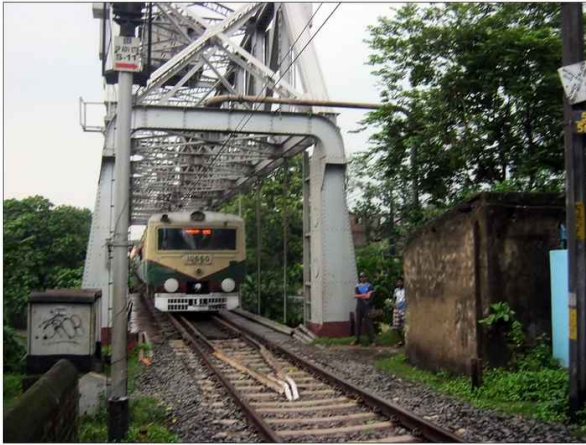
The Lock Gate bridge. Confluence of Belaghata Canal & the river.
