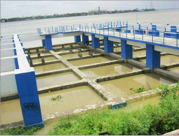
KMC Water Treatment Plant @ Baghbazar Outer
